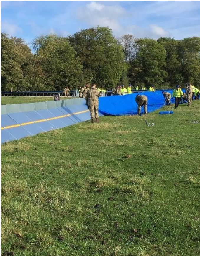
Photo from exercise to practice deployment of temporary flood barriers in Weybridge 2018.
