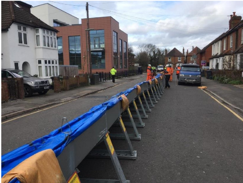
Barrier deployed in Guildford before expected flooding in 2020
